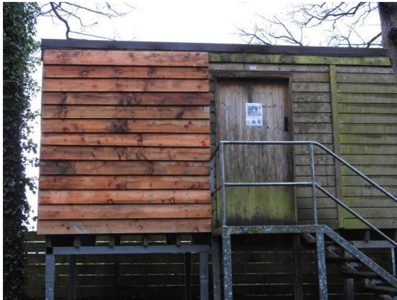
Plate 5.4 Bat panel (left of the door) on the bird hide at Ballygilgan Nature Reserve.
